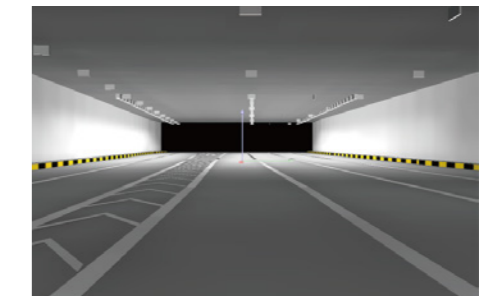
Asymmetric against-glare lighting, suitable for horizontal installation of lighting in tunnels
